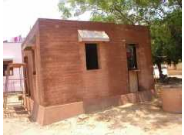
A Model House for Anumandhai Kuppam SHGs - under Construction
